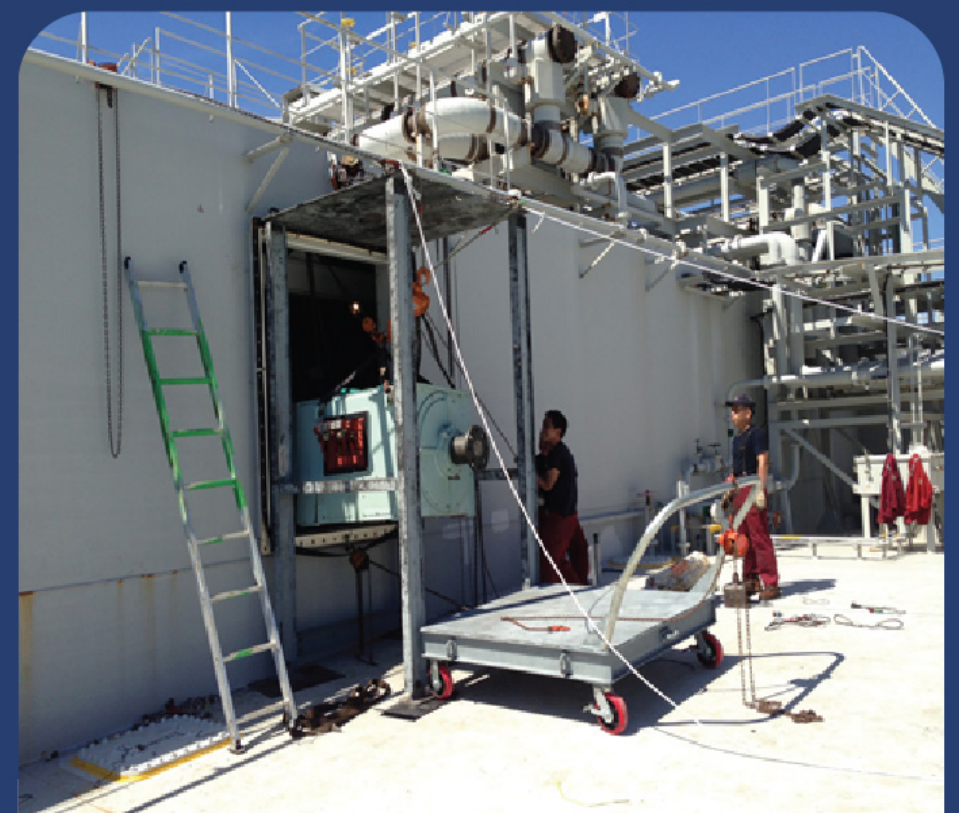
DISMANTLING COMPR MOTER 440V 230KW 12POLE 585RPM
