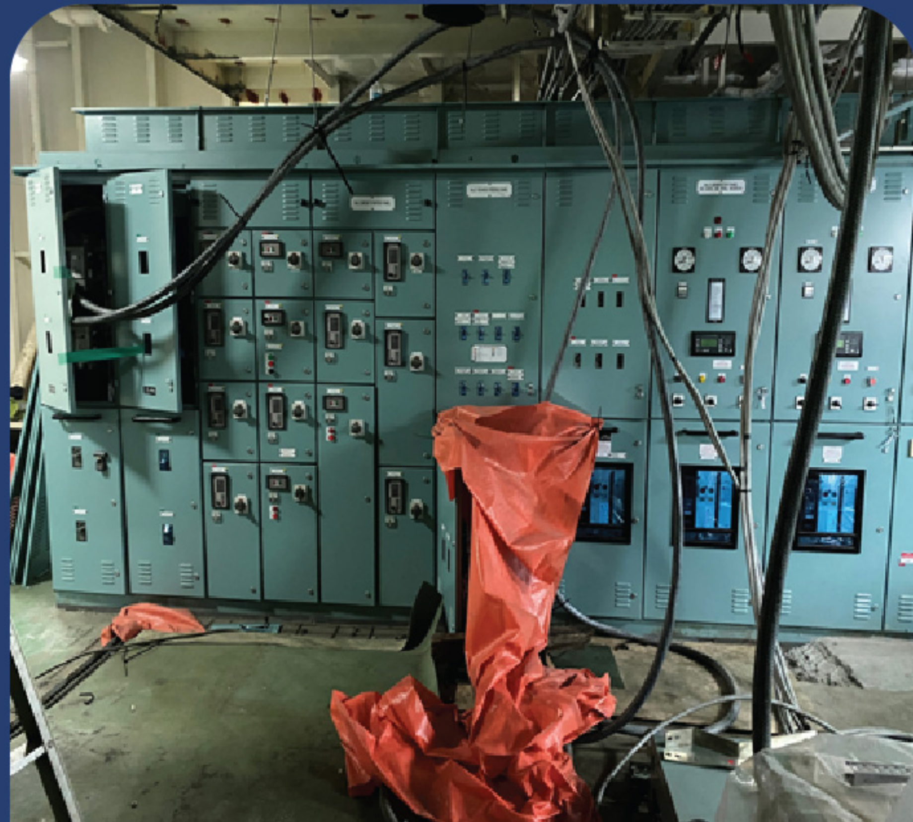
RETROFIT OF MSBD, ESBD & G/E SYSTEM CHECKING
