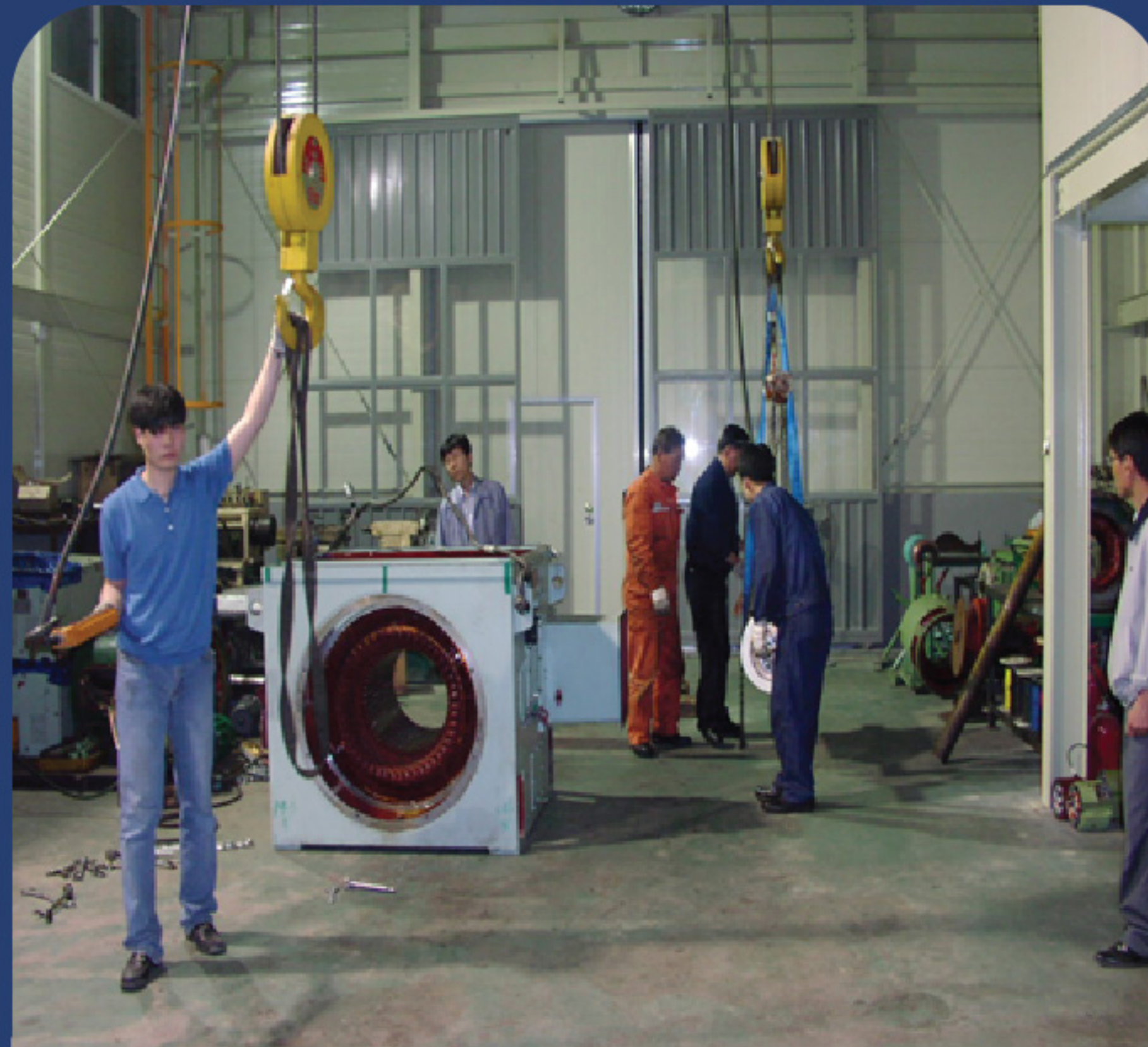
OVERHAUL H.P COMP. MOTOR TO REPAIR ROTOR SHAFT DAMAGE
